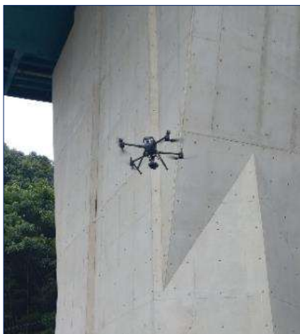
[ UAVを用いた橋梁点検 ]
