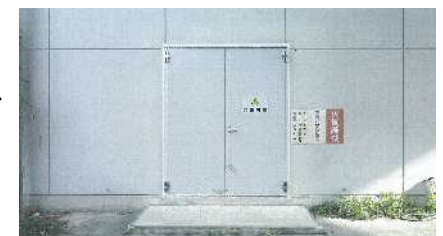
[宇品電気室防水扉(完成)]
